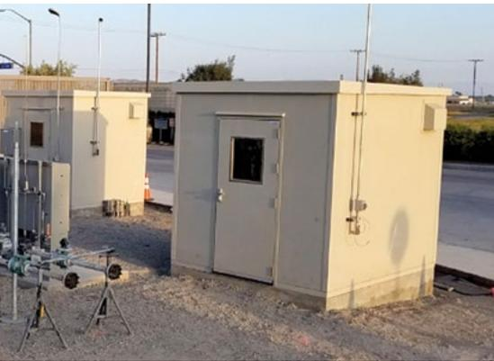
**Biogas is conditioned at the CR&R anaerobic digestion facility in Perris (CA) and then transported about 1.4 miles via a high-pressure steel pipe (top) to the SoCalGas interconnection “point of receipt” (above). The gas utility monitors the RNG quality at this location, and then meters and odorizes the volume of RNG put into its pipeline network.**
